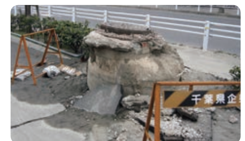
2011: Great East Japan Earthquake; damage to a manhole in the Takasu District, Urayasu City (Institute of Scientific Approaches for Fire & Disaster)
