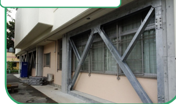
After seismic reinforcement works
