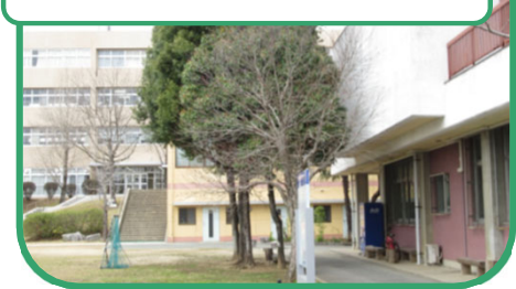
Before seismic reinforcement works
