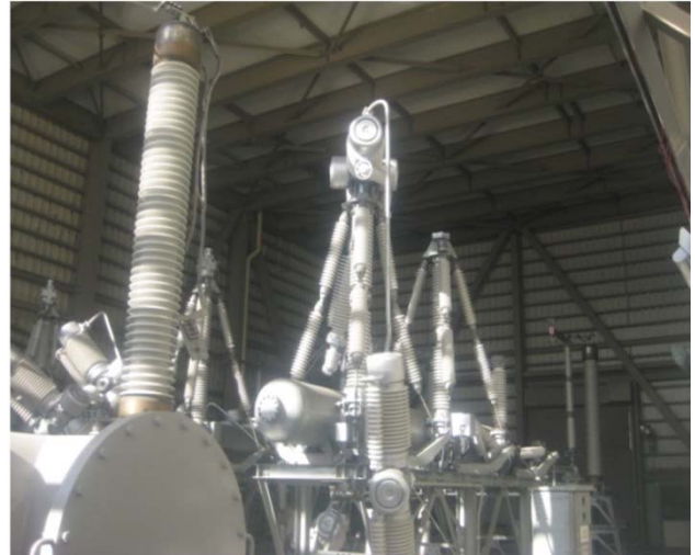
March 23, 2011 Photographed by Tokyo Electric Power Company Picture (ii): Breaker (O-82) having fallen inside the switching station for Units 1 and 2.
