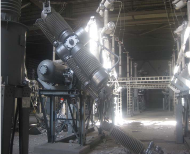
March 23, 2011 Photographed by Tokyo Electric Power Company Picture (i): Breaker (O-81) having fallen inside the switching station for Units 1 and 2.
