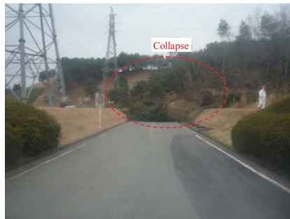
Although this is not an emergency access road, the slopes collapsed and blocked the road, leaving it impassable. Photographed by TEPCO on March 20, 2011
