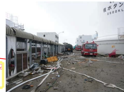
Although no particular problem was observed with the road, rubble scattered around due to the tsunami and explosion Photographed by TEPCO on March 16, 2011
