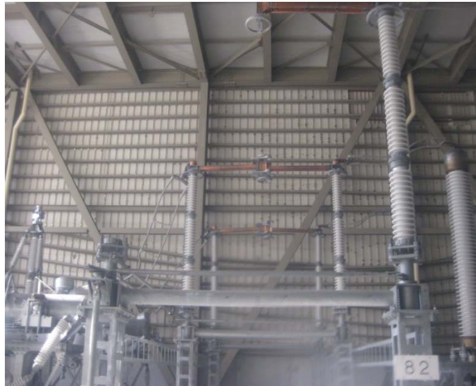
March 23, 2011 Photographed by Tokyo Electric Power Company Picture (iii): Disconnection switch having fallen inside the switching station for Units 1 and 2.
