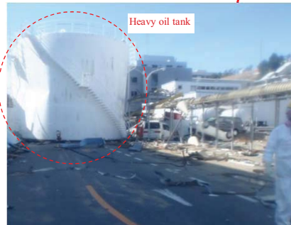
Although there was no major damage to the road, a heavy oil tank washed in by the tsunami. No particular problem was observed on the straight road stretching from the main gate road, leaving it impassable. Photographed by TEPCO on March 17, 2011
