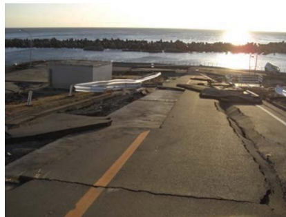
Although this area had had reinforcement work, cracks and gaps occurred on the sides of road which had not been reinforced. Photographed by TEPCO on March 17, 2011
