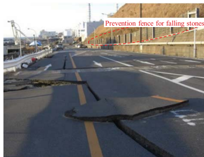
The lane on the sea side cracked parallel to the road and created a gap. The west side was passable. Photographed by TEPCO on March 17, 2011.
