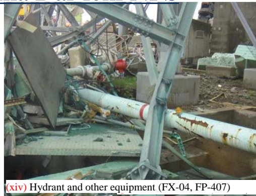
(xiv) Hydrant and other equipment (FX-04, FP-407) August 25, 2011 Photographed by Tokyo Electric Power Company
