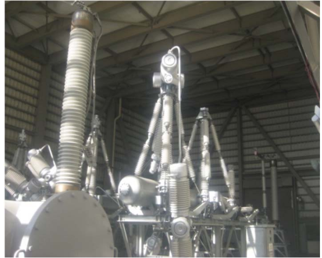
March 23, 2011 Photographed by Tokyo Electric Power Company Picture (ii): Breaker (O-82) having fallen inside the switching station for Units 1 and 2.
