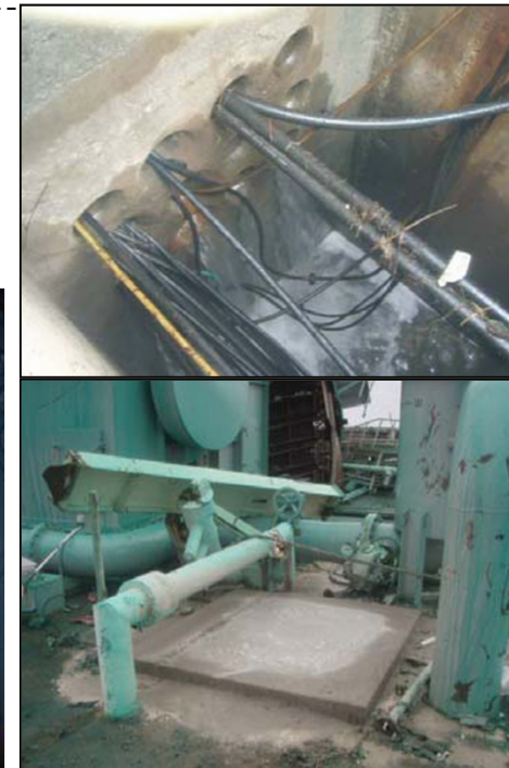
Above: water flow to the power supply cable pit (photo by TEPCO at 10:30 on May 11) Below: after concrete injected into the pit where leakage found (photos by TEPCO at 17:30 on May 12) Prepared by TEPCO.
