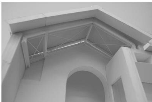
(2) Reinforcement of the roof structure plane of the Storage 1 (former fan room) side bay, looked up from the passage between the two buildings
