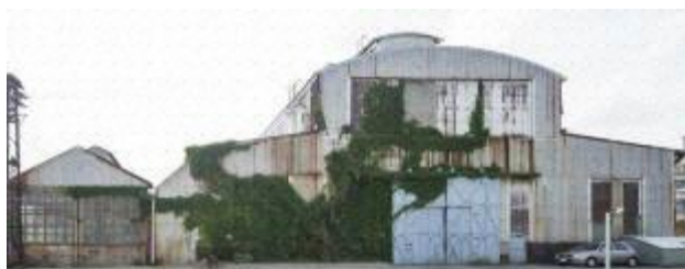
Repair Shop (west side exterior view)
