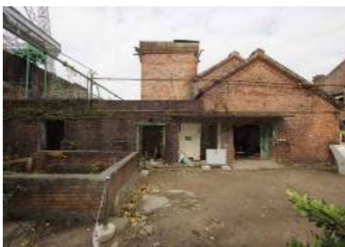
Figure 4 Storage and Pumping Station
