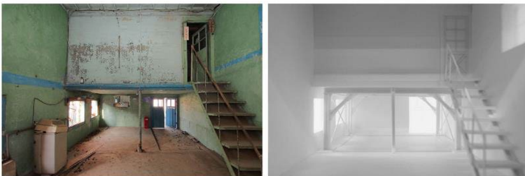
(e) Falling prevention device under the drying room viewed from the changing room
