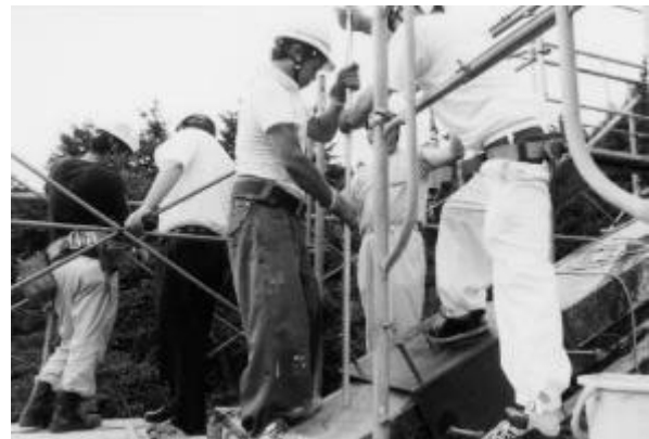
Insert a reinforcing bar (brick width: 333 mm, 1-D22)
