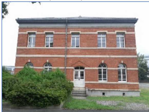
Exterior view (west side)
