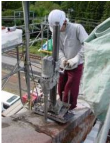
Drill a reinforcing bar insertion hole (42 \phi , 3.8–7.0 m)
