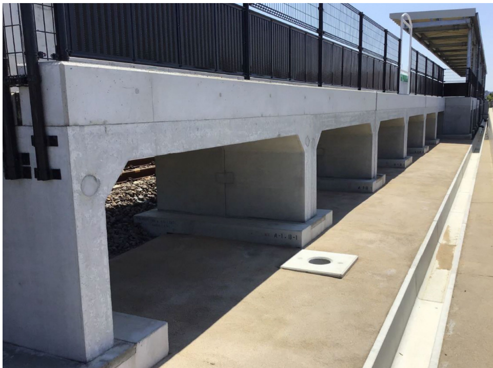
Figure 6. Example of a Platform built using a gate-type culvert structure (Proposed Structure)
