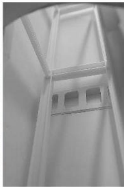
(a)(b) Exhaust tower frame reinforcement looked up at from just under the tower
