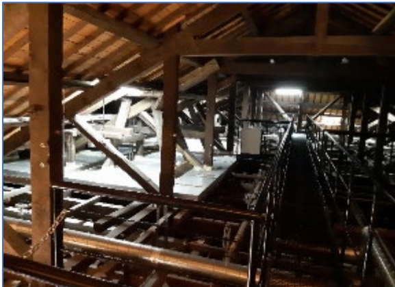
Attic (inspection corridor, waterproof pan, etc.)
