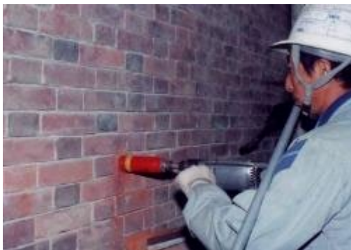
1. Chip away bricks deteriorated more than half
