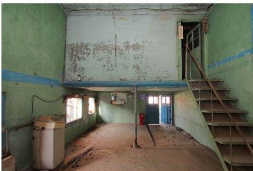
(e) Falling prevention device under the drying room viewed from the changing room
