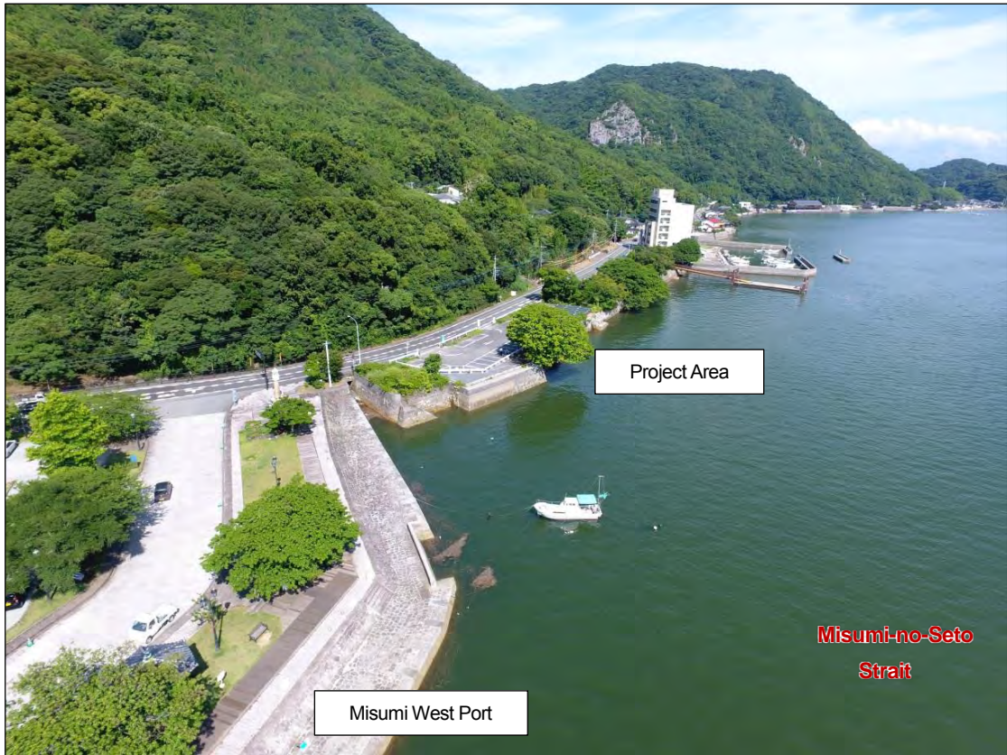
Figure 4 Present state of project area (aerial view of the buffer zone and floating pier from above the component part)
