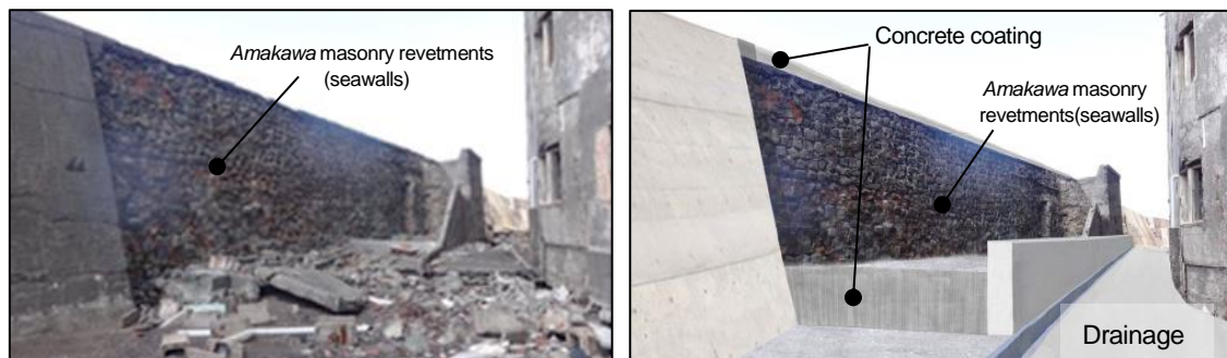
Figure 7: Images of seawall revetments conserved by Option 1 (left: before conservation; right: after conservation)
