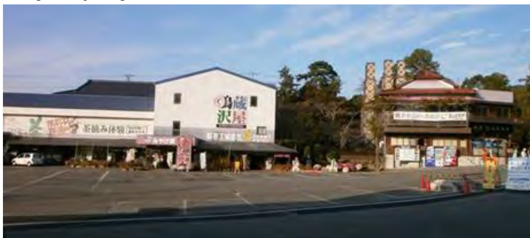
Before construction (November 2014)
