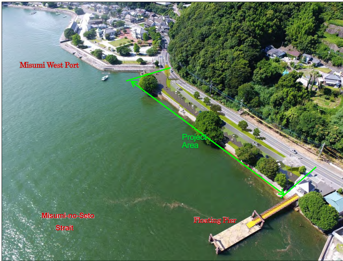
Figure 7 Completed project image (aerial view of buffer zone and Misumi West Port from above the floating pier)
