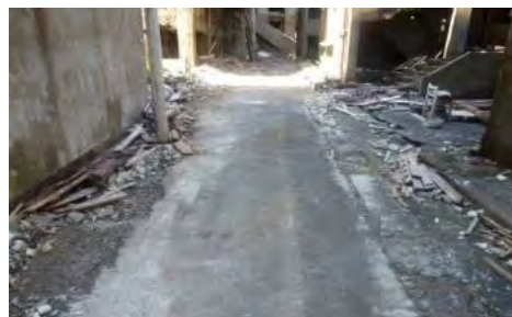
Figure 11: Current site management passage
