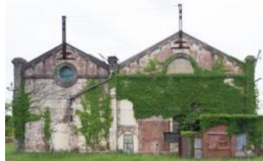
Onga River Pumping Station (view of west side)
