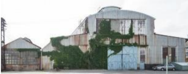
Repair Shop (view of west side)
