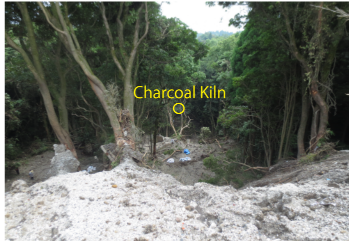
(3) View from upper part of landslide (photographed July 9, 2019)
