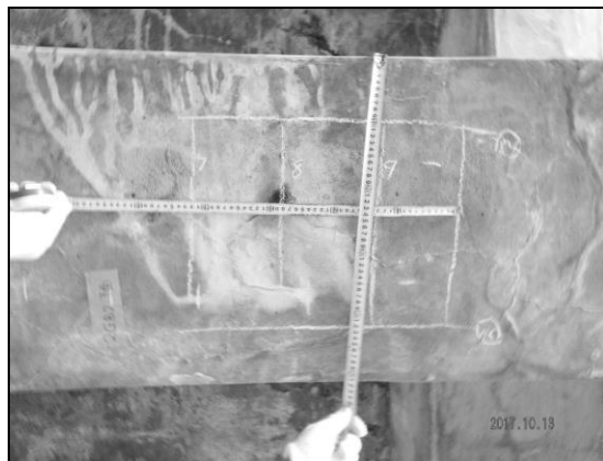
Rebar arrangement at bottom of beams
