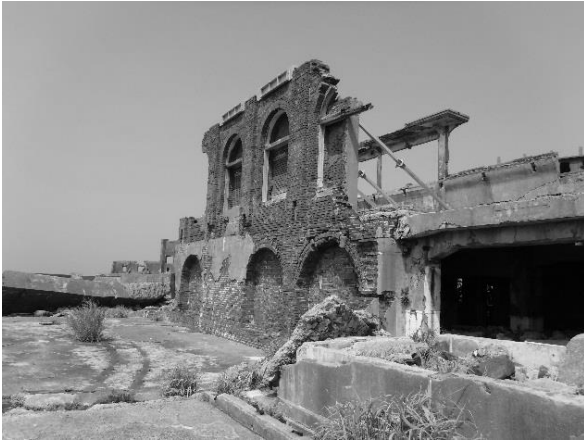
Surveyed building, outside (Eastern side)
