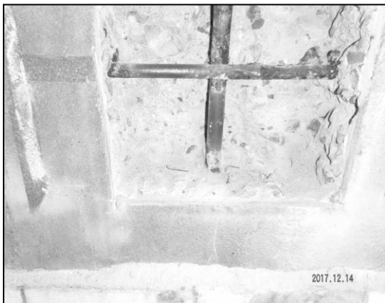
Rebar conditions (column)
