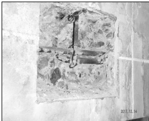
Rebar conditions (beam)
