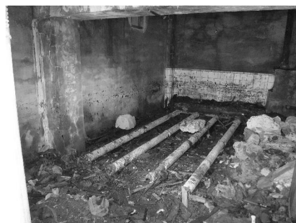
Surveyed building, inside (Warehouse)
