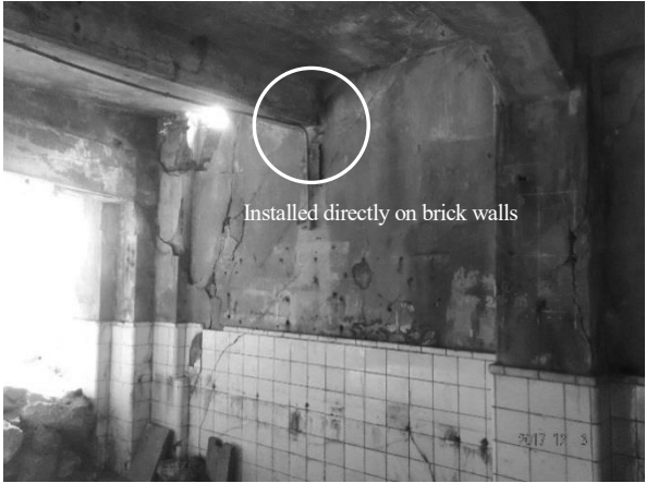
Photo 2-4-106. Joint condition between Beam B5 and brick walls
