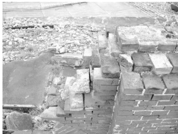
Photo 2-4-109. Western side of brick walls
