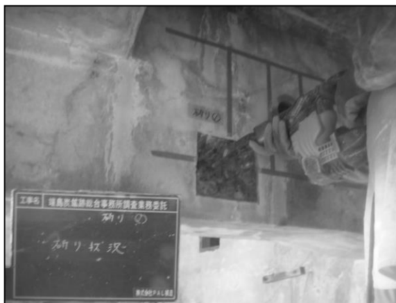
Concrete chipping work
