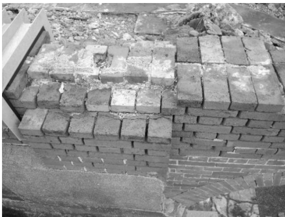
Photo 2-4-108. Top of brick walls
