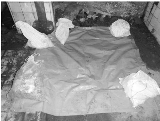
Photo 2-4-80. Exploratory Drilling Site ①, backfilling completed
