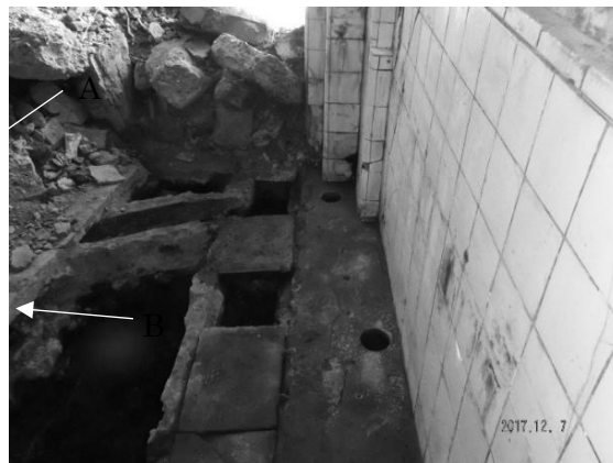
Photo 2-4-104. Core boring site; on base lines A and 3 intersection
