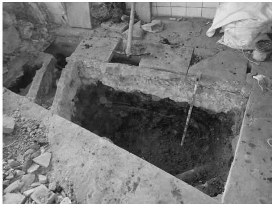
Photo 2-4-93. Exploratory Drilling Site ②, drilling completed; viewed from south
