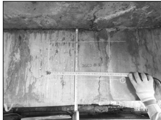
Examining bar arrangement (2GC2, side)
