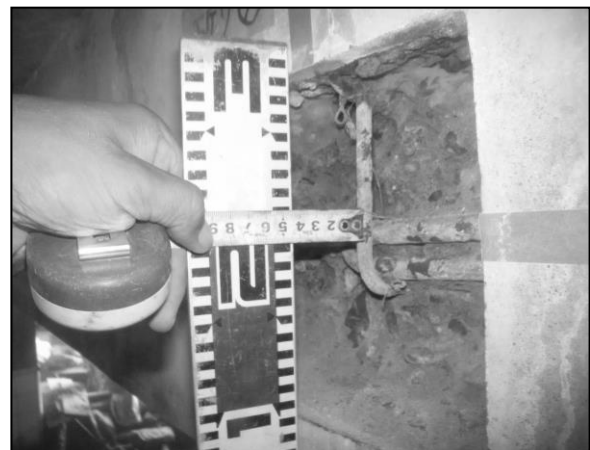
Measuring concrete cover thickness
