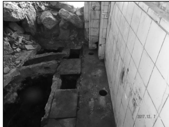
After a core has been drilled out
