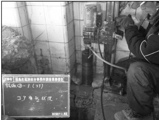
Drilling out a core
