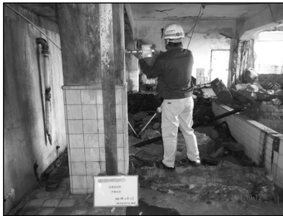
Photo 2-4-71. Performing rebound hammer test
