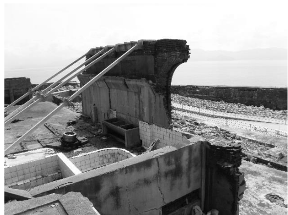
Surveyed building, outside (Western side)
