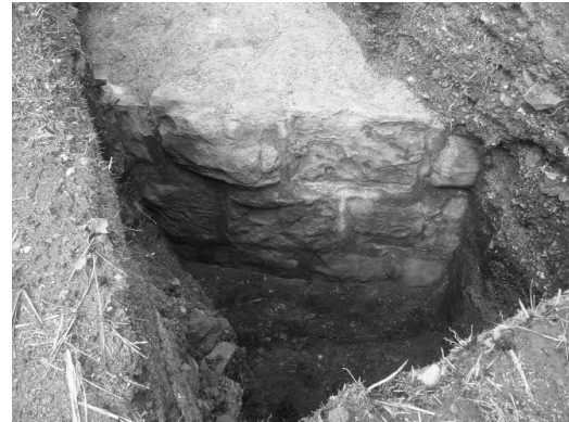
Photo 2-3-94. Trench No. 2, stone seawall
