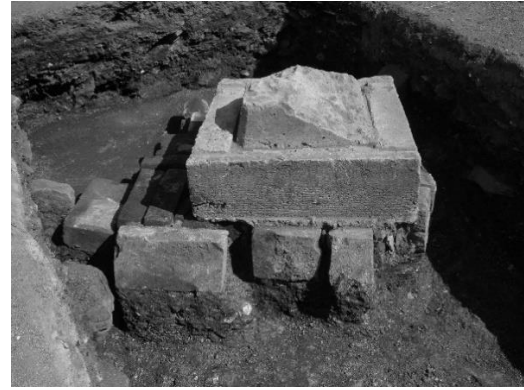
Photo 2-3-98. Trench No. 4, remains of foundation
