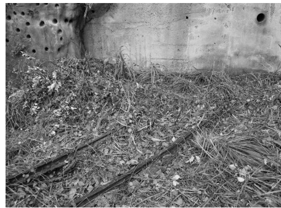
Photo 2-3-57. Mouth of Pit survey 2; Tram tracks
