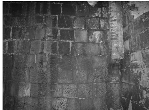
Photo 2-3-86. Pit No. 3, western wall
