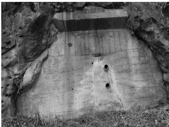
Photo 2-3-56. Mouth of Pit survey 2; Full view
