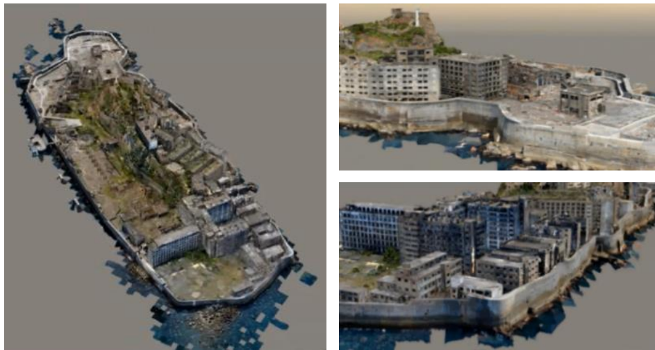
Figure 4. 3D model of Hashima Coal Mine made from 3-D laser survey
