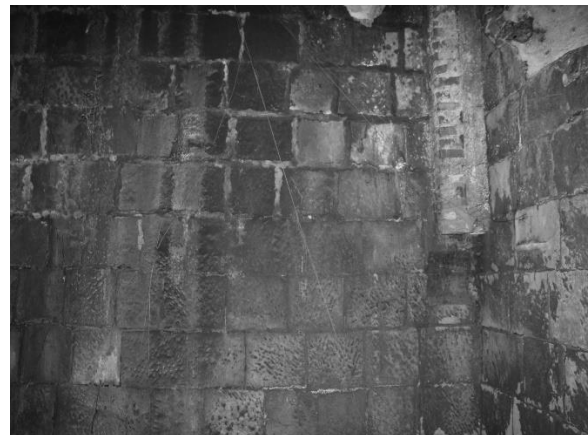
Photo 2-3-86. Pit No. 3, western wall
