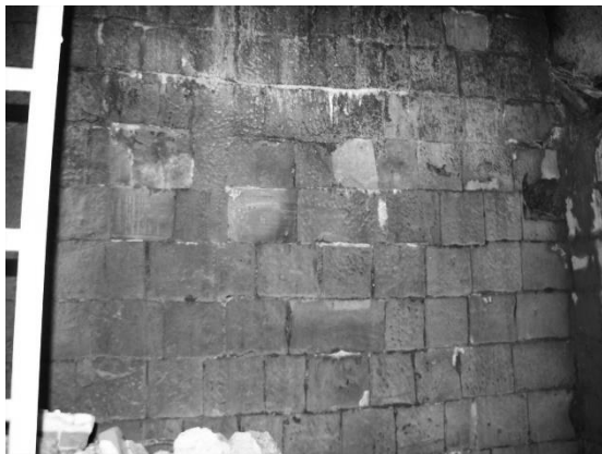
Photo 2-3-67. 3-E37_Eastern wall, lower parts
