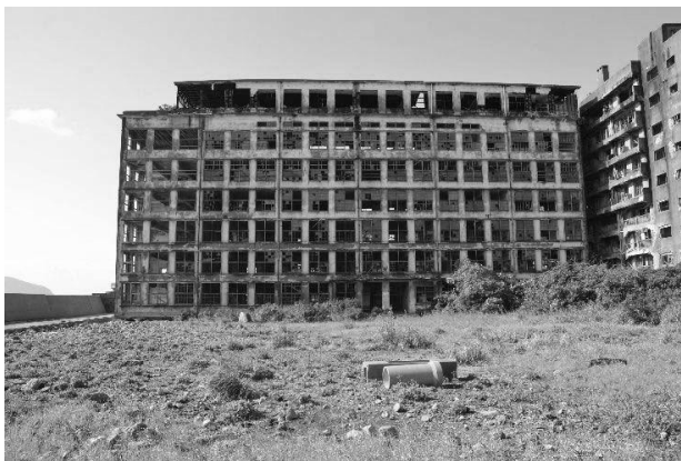
North side front view
