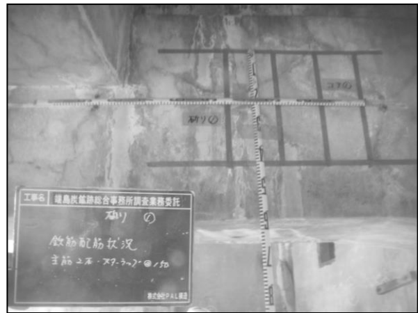
Rebar arrangement
