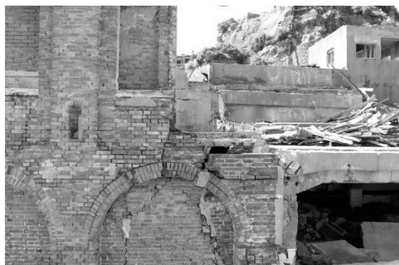
Photo 2-4-110. Eastern side of brick walls
