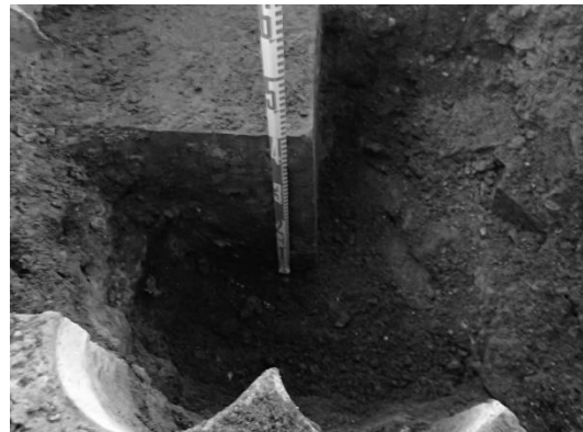
Photo 2-4-75. Exploratory Drilling Site ①, survey underway
