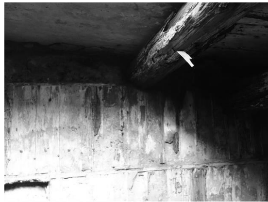
Photo 2-3-68. 3-A04_Eastern wall, upper parts
