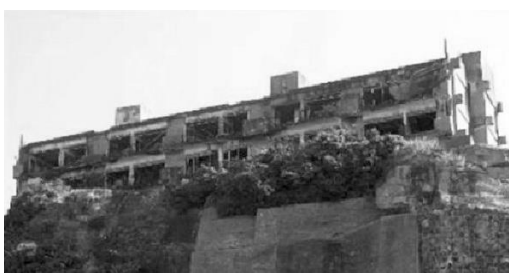
Photo 2-4-122 Building No.3 appearance
