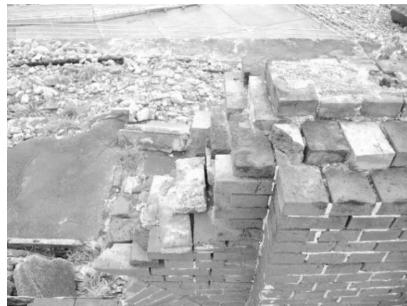
Photo 2-4-109. Western side of brick walls
