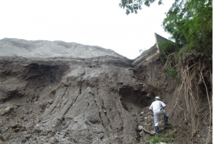
(1) Upper part 1 of landslide (photographed July 9, 2019)
