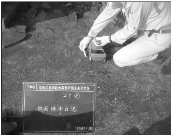
Rebar exploration (electromagnetic wave radar method) work
