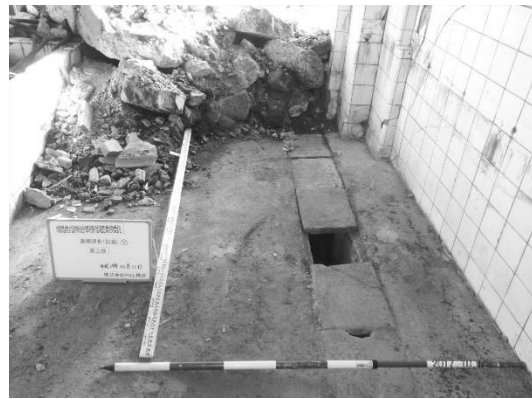
Photo 2-4-77. Exploratory Drilling Site ②, before start
