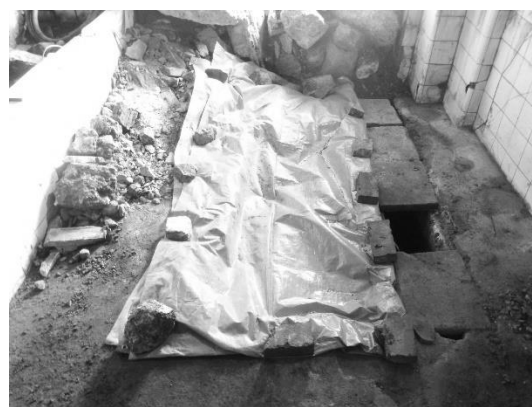
Photo 2-4-81. Exploratory Drilling Site ②, backfilling completed
