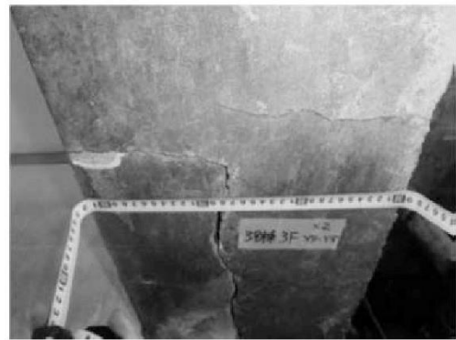
Photo 2-4-123 Beam dimension measurement
