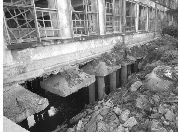
Building No.70 foundation
