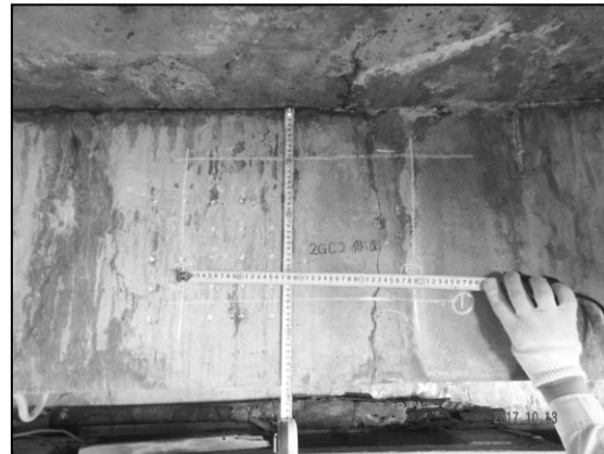
Examining bar arrangement (2GC2, side)
