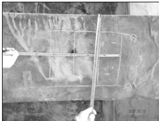
Rebar arrangement at bottom of beams
