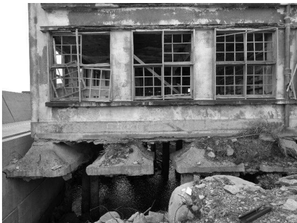
Foundation on the north side of the building
