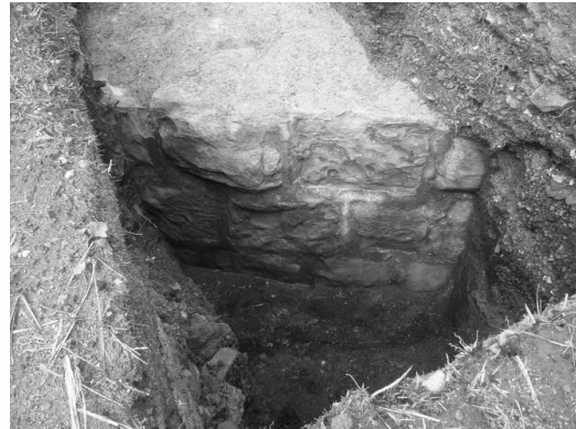
Photo 2-3-94. Trench No. 2, stone seawall
