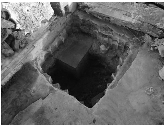
Photo 2-4-84. Exploratory Drilling Site ①, drilling completed
