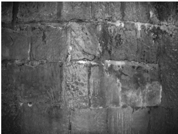
Photo 2-3-85. Pit No. 3, eastern wall
