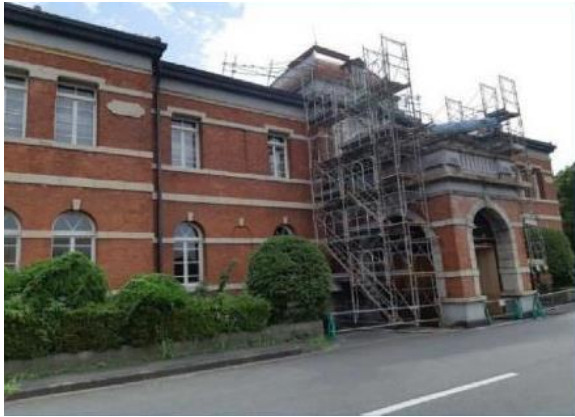
Exterior view (north side)
