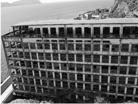
Building No.70 appearance
