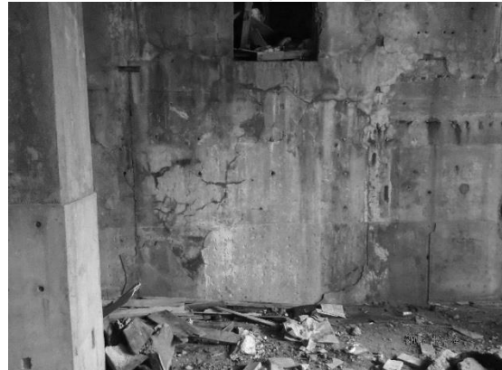
Photo 2-4-96. Plane A (North), outer wall
