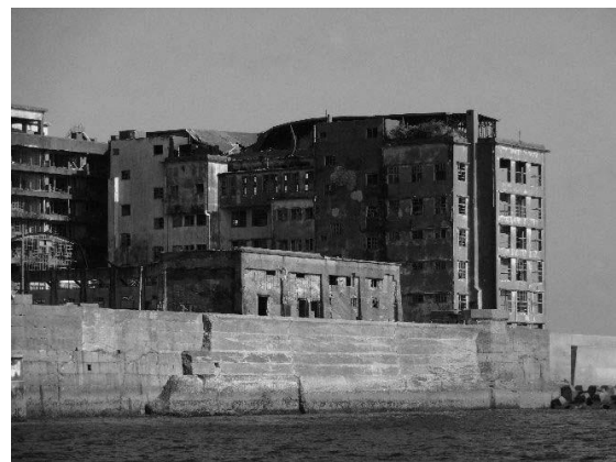
From the southeast side
