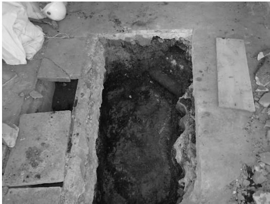
Photo 2-4-78. Exploratory Drilling Site ②, survey underway
