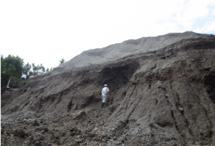
(2) Upper part 2 of landslide (photographed July 9, 2019)
