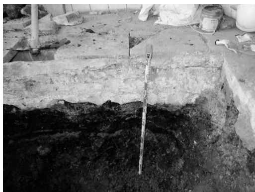
Photo 2-4-86. Exploratory Drilling Site②, Southern wall
