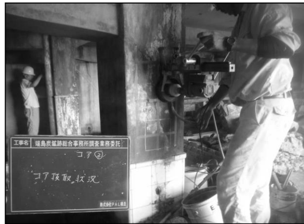
Core drilling work
