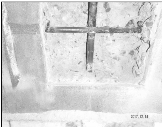
Rebar conditions (column)
