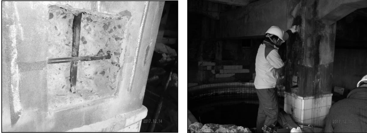
Photo 2-4-72. Measuring reinforcement corrosion degree
