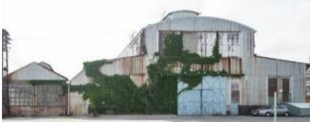
Repair Shop (view of west side)
