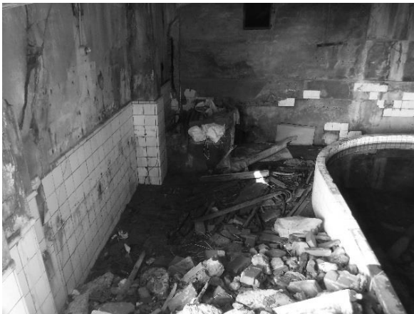
Surveyed building, inside (Bath)
