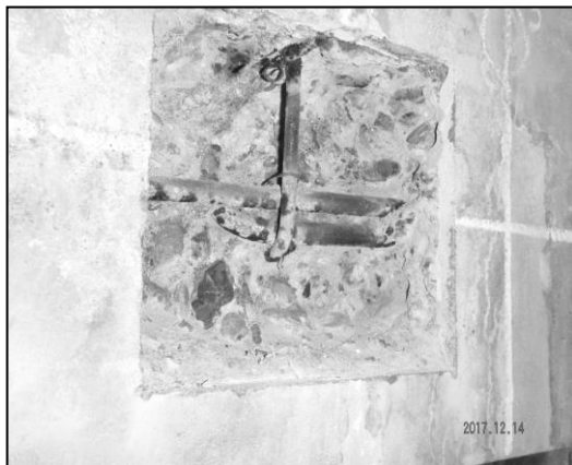
Rebar conditions (beam)
